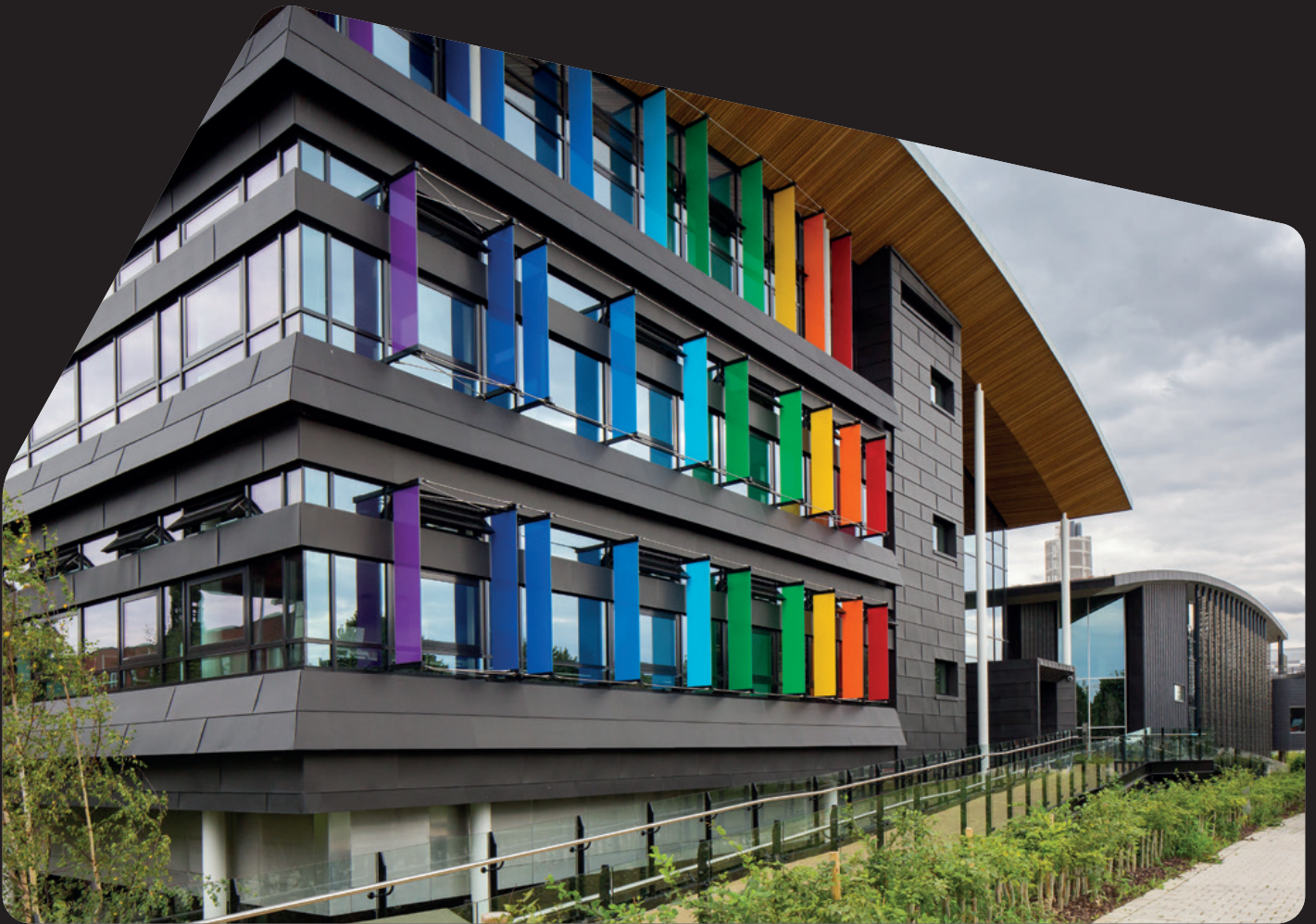
BREEAM: Universiteit van Cambridge Maxwell Centre - Architect: Building Design Partnership (BDP) - Cambridge (Royaume-Uni)
