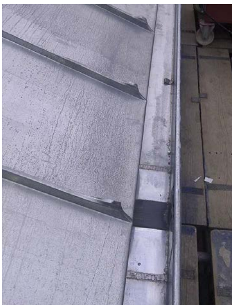
Expansion joint soldered to gutter
