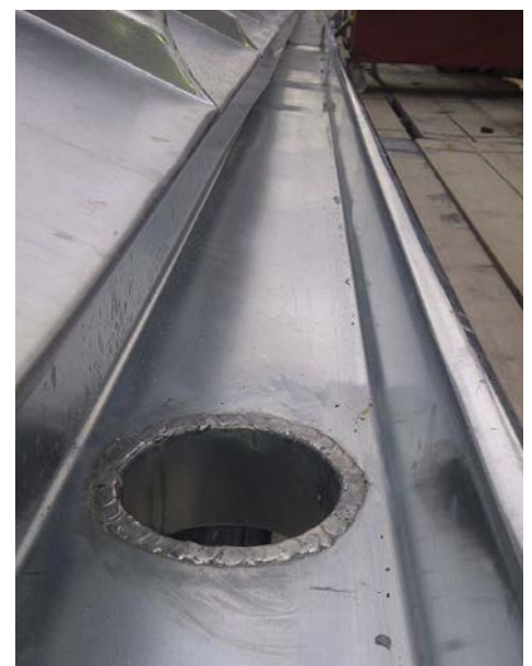
Downpipe outlet starter soldered to gutter
